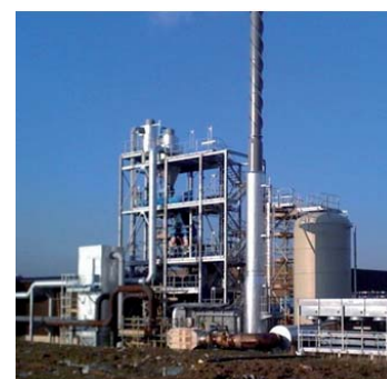
Fully Constructed Plant
